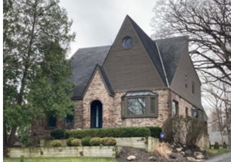
The steeply pitched gable and the rounded arch are common on Tudor Revival style houses. Photo by KDG, 2023.
