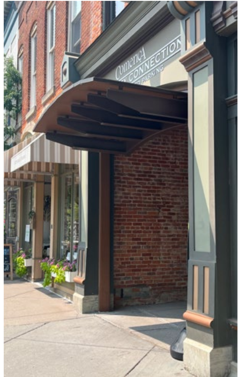
The awning pictured above is not appropriate as the shape and materials used are not compatible with the historic character of the district. Photo by KDG, 2023.
