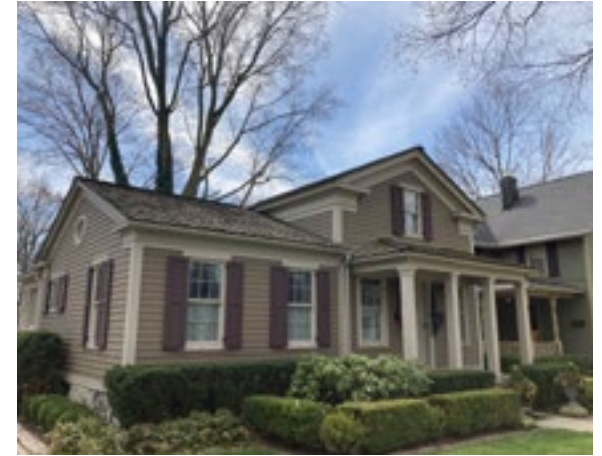
The pediment trim and gable returns are both features of the Greek Revival style. Photo by KDG, 2023.
