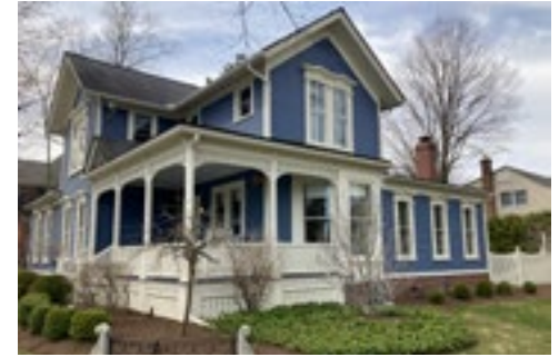
This house dates to 1860 but the porch shown here was not added until 1900. This is a good example of an architectural feature that has gained significance over time even though it's not original to the building. Photo by KDG, 2023.
