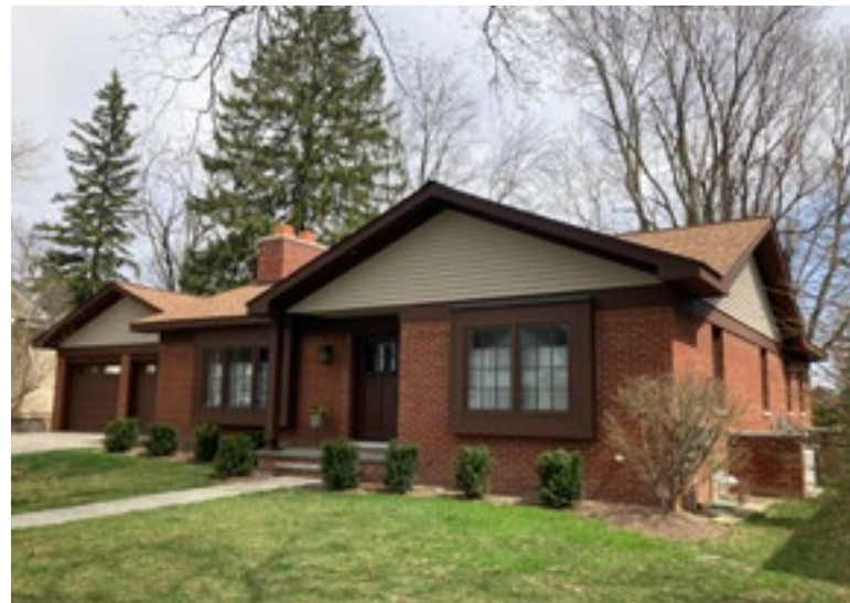
This house has typical Ranch stylistic details including multiple cladding materials, moderately overhanging eaves, and a connected garage. Photo by KDG, 2023.
