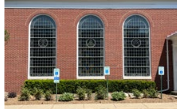
While the First Presbyterian Church is a non-historic resource in the historic district, the HDC still has the authority to review exterior changes to ensure alterations do not detract from the surrounding historic resources. Photo by KDG, 2023.
