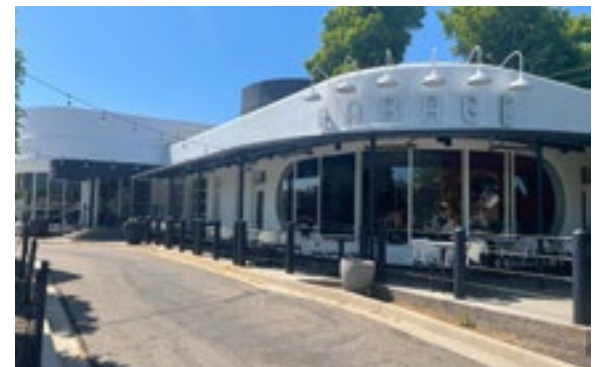
Special care is required to arrange mechanical equipment on roofs above single story commercial buildings so that the equipment is not visible from the right-of-way. Photo by KDG, 2023.
