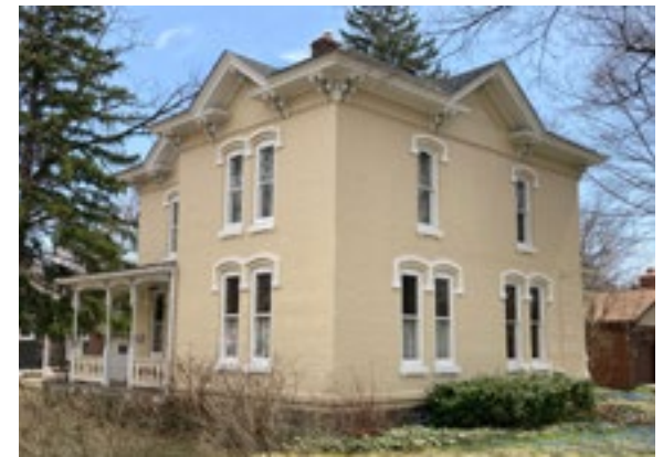
The window hoods, bracketed cornice and one-story porch are indicative of the Italianate style. Photo by KDG, 2023.
