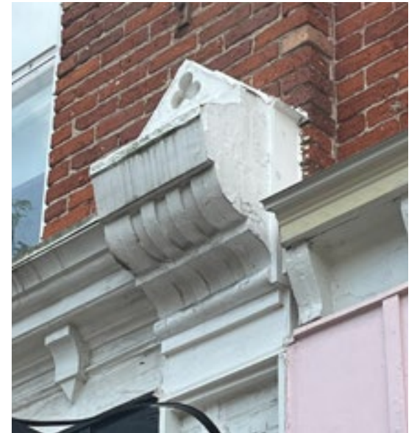
On commercial resources, wood exterior wall materials are typically used as ornament on the building and storefront, as pictured here. Photo by KDG, 2023.
