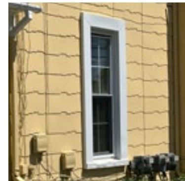
It is not appropriate to replace historic wood windows with vinyl units and vinyl trim. Photo by KDG, 2023.
