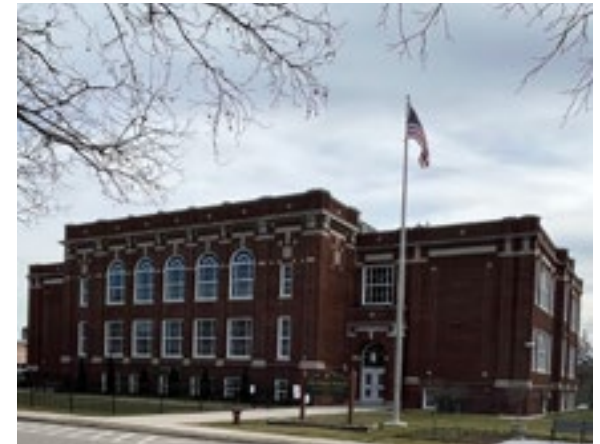
Preserving important places like the Old Village School enhances the community by connecting residents to the past. Photo by Leanie Bayly.
