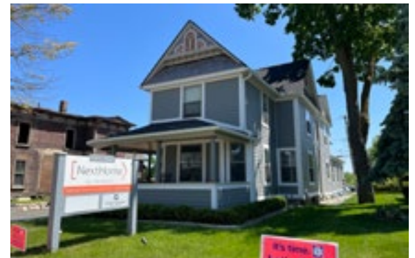
Located just east of the commercial heart of Northville, this residence has been adaptively reused as a place of business. Photo by KDG, 2023.
