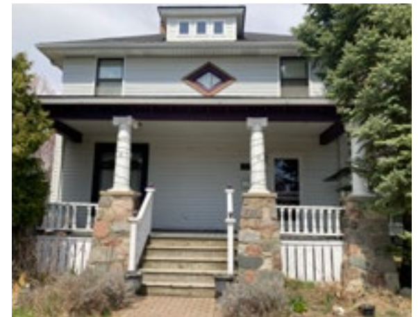
The battered (tapered) stone columns, centrally placed attic dormer, hipped roof, and full width porch are all common on Prairie style homes and homes with Prairie style elements. Photo by KDG, 2023.
