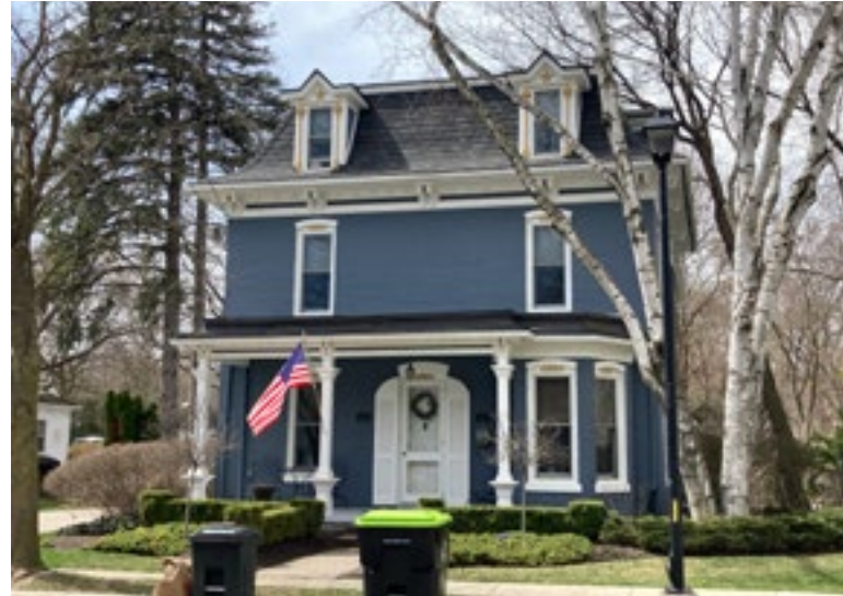
The mansard roof, dormers on the lower roof slope, and the bracketed cornice are all indicative of the Second Empire style. Photo by KDG, 2023.
