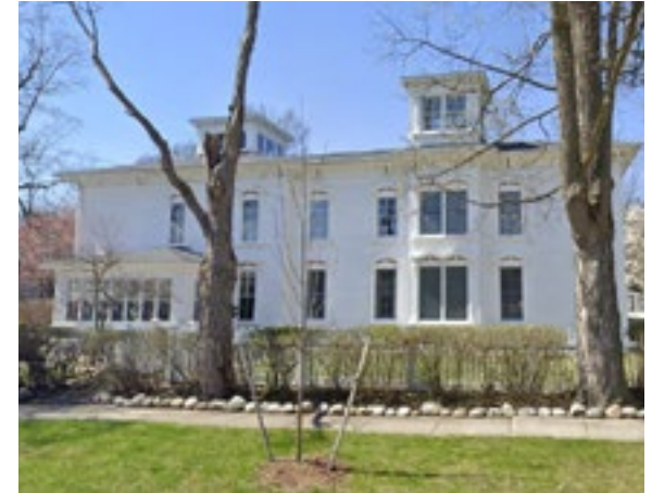
It is not appropriate to construct a large addition (shown at right) that is indistinguishable from the original house as it uses the same general roof line, cornice line, wall plane, siding lap, window surrounds, and ornamentation. Photo by KDG, 2023.
