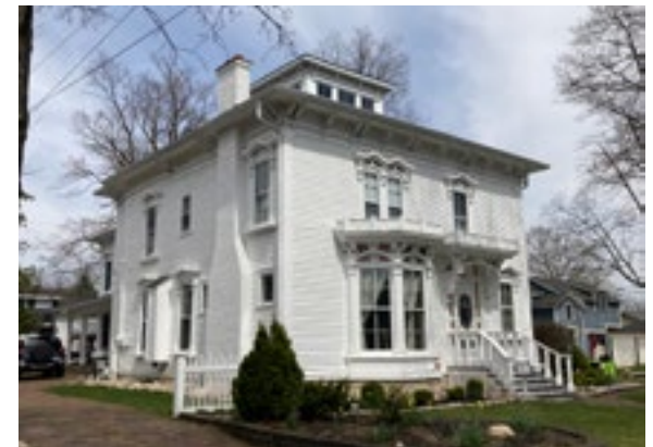
The cupola, centered on the roof, is common in the Italianate style. Photo by KDG, 2023.
