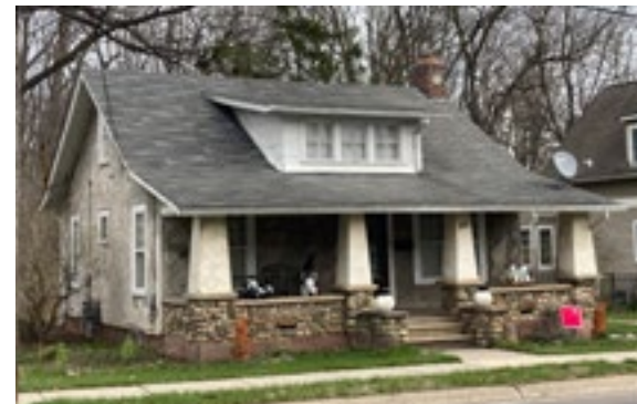
This Craftsman features battered (tapered) columns, a stone porch, and stucco cladding. Photo by KDG, 2023.
