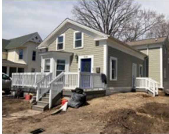
The gable returns seen here are a typical feature on Greek Revival houses. Photo by KDG, 2023.
