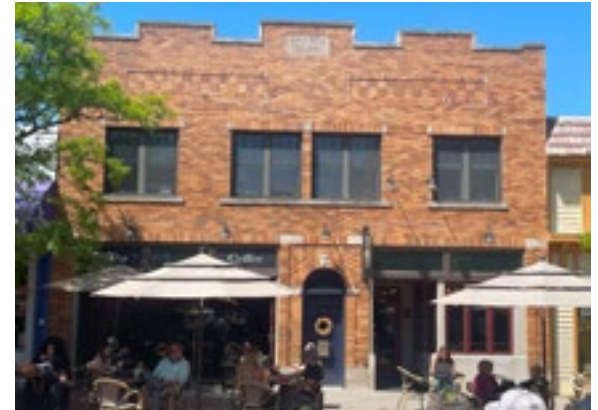
It is appropriate for rooftop mechanical equipment to be situated so that it is not visible from the public right-of-way. Rooftop mechanical equipment is not visible on these buildings within Northville's historic district. Photo by KDG, 2023.
