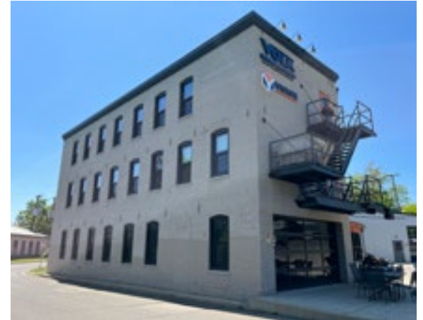
Through adaptive reuse, this late 1800s industrial building has become office space for local business. Photo by KDG, 2023.
