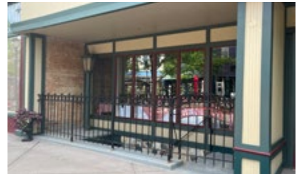
The alteration of the storefront's relationship to the sidewalk, through the addition of an exterior stairway, is not appropriate as the stairway disrupts how the storefront interacts with the sidewalk. Photo by KDG, 2023.
