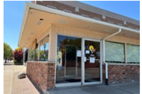
While most of Northville's commercial buildings date to the late-nineteenth and early-twentieth centuries, mid-twentieth century architecture should not be overlooked. Materials like aluminum are more common on exterior doors from this era. Photo by KDG, 2023.
