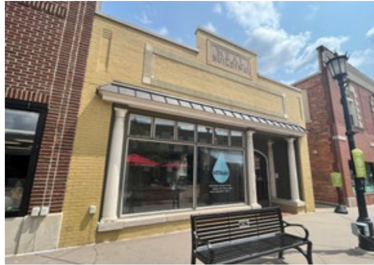
This single story commercial building highlights the Commercial style with the stepped parapet, recessed entry, and decorative brickwork near the cornice. Photo by KDG, 2023.
