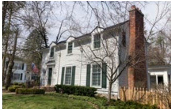
This side gabled Colonial Revival style home features six-over-twelve windows and classically detailed pilasters around the main entrance. Photo by KDG, 2023.
