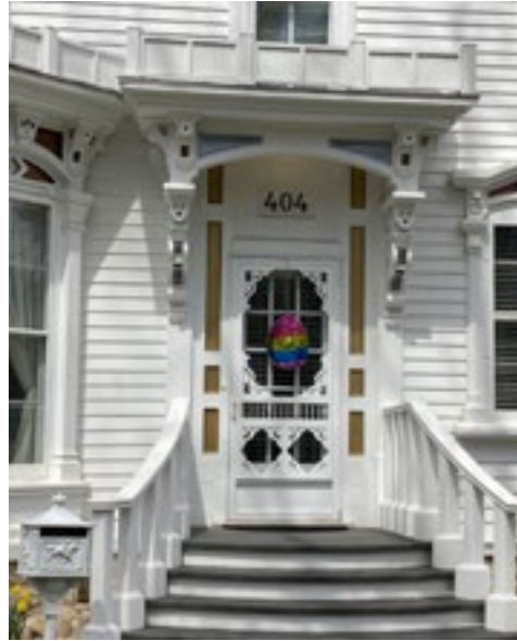
Historic doors often feature elaborate entry surrounds like seen here. This door surround is an important part of the door and should be preserved. Photo by KDG, 2023.
