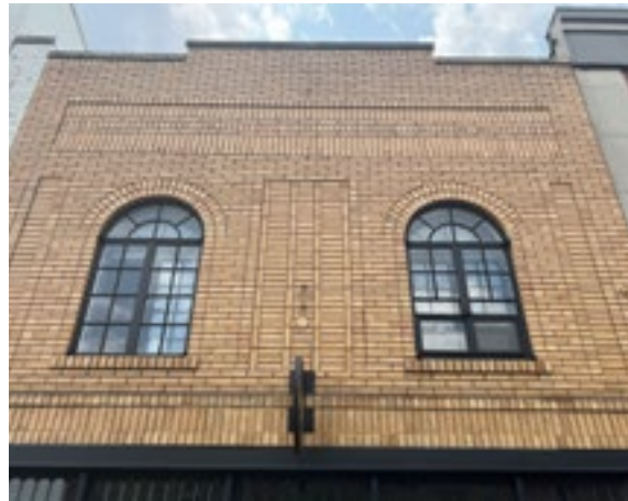
Preservation of exterior materials includes preserving the pattern and arrangement of historic materials, such as the varied brick bonding patterns used on this façade. Photo by KDG, 2023.
