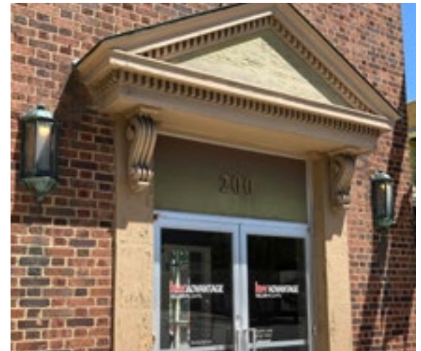
Typical exterior lighting in Northville's historic district. Photo by KDG, 2023.
