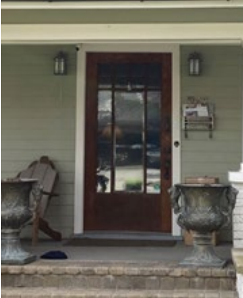
The width of this door and the beveled glass are character defining features of this historic door. Photo by KDG, 2023.
