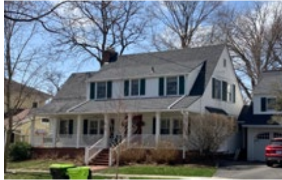
Built in 1930 and typical of the style, this Colonial Revival home features paired windows at the first floor with eight-over-eight sashes and a centrally placed main entrance. Photo by KDG, 2023.
