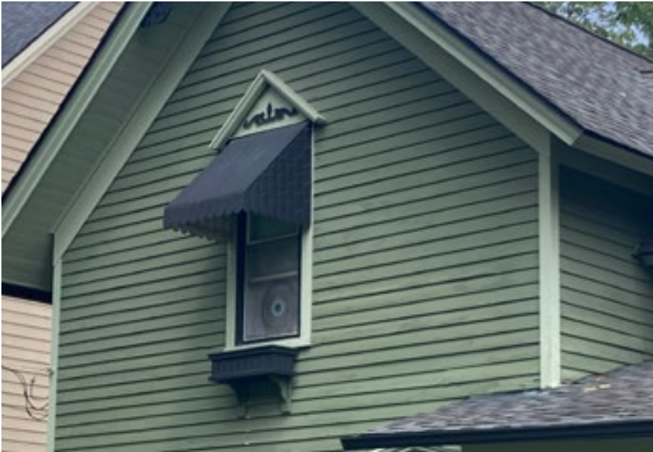
Appropriate wood siding has a narrow reveal and intersects with corner boards and window frames. Photo by KDG, 2023.
