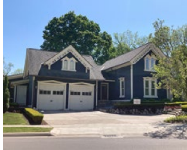
It is appropriate that attached garages only be located on facades that are minimally visible from the right of way. Highly visible and too large in scale, attached garages like this are not appropriate. Photo by KDG, 2023.
