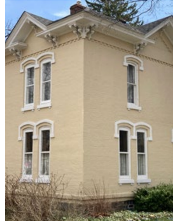
It is not appropriate to paint brick that was historically unpainted. Photo by KDG, 2023.
