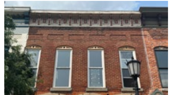
Painting schemes that highlight architectural ornament and features are compatible with the historic character of many of the commercial buildings within Northville's historic district. Photo by KDG, 2023
