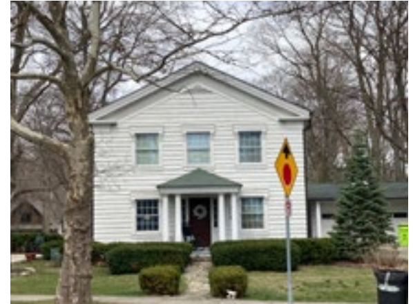
Greek Revival style. Photo by KDG, 2023.
