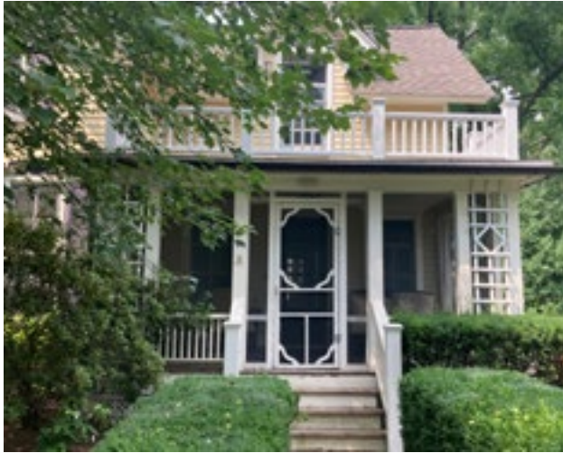
Enclosing a porch with screens is appropriate only for secondary or rear facades. Photo by KDG, 2023.
