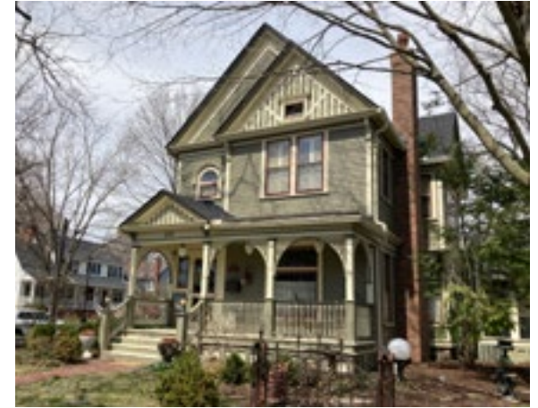
This Queen Anne style home has elements of the Stick sub-type with applied stickwork in the gable eave. Photo by KDG, 2023.
