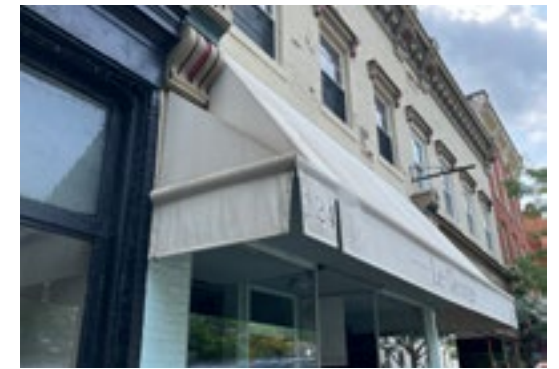
Triangle-shaped awnings with loose valances are historically compatible with the historic district and are therefore appropriate. Photo by KDG, 2023.
