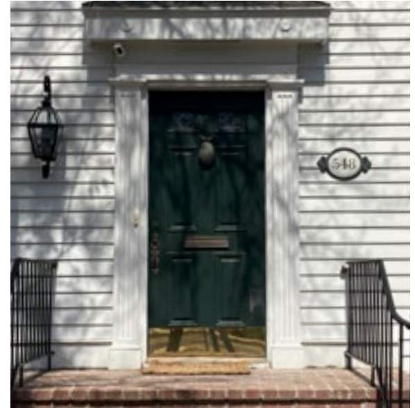
Historic hardware such as the door handle, letter box, and door knocker contributes to the character of the historic door. Photo by KDG, 2023.
