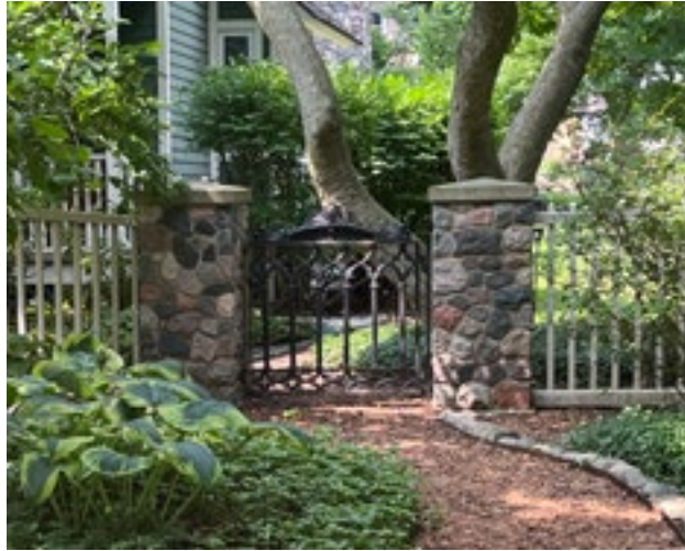
Historic fencing and fence posts should be preserved and maintained. Photo by KDG, 2023.
