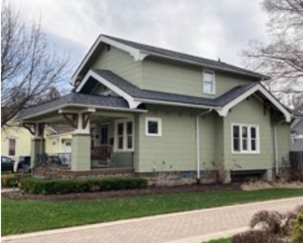
Large second story additions are not appropriate if highly visible from the right of way like this. Photo by KDG, 2023.
