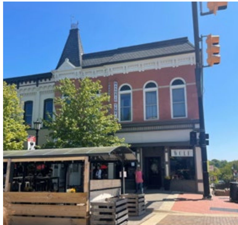
The mansard roof, prominent tower feature on the roof, bracketed cornice, and round arch windows indicates the Second Empire style. Photo by KDG, 2023.
