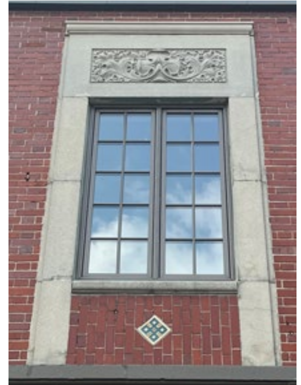
The cast stone and decorative tile add to the beauty and historic character of this building. Photo by KDG, 2023.
