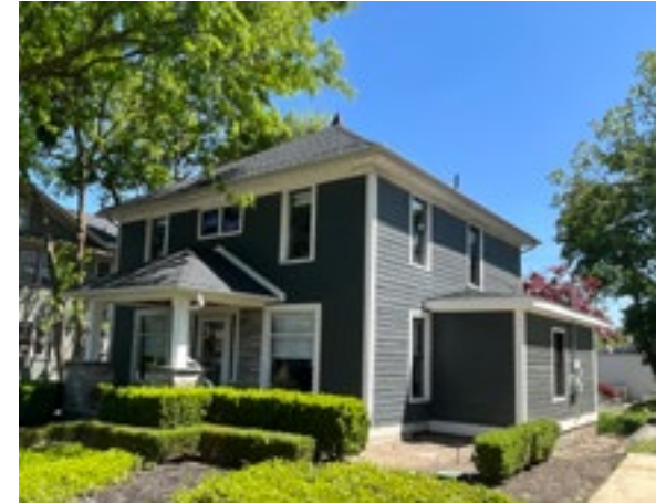
This Prairie style Foursquare still features its pyramidal roof, but most other historic features (including windows and siding) have been removed or covered over. Photo by KDG, 2023.
