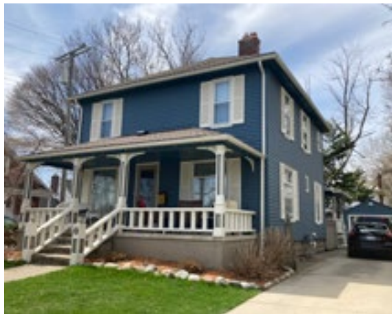
A Prairie style Foursquare with full width front porch and pyramidal roof. Photo by KDG, 2023.
