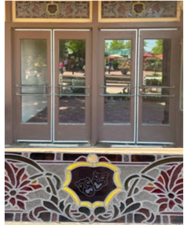
The preservation of the historic doors, hardware, stained glass transoms, and trim maintains the historic character of Northville's theater. The transoms located above the doors contain stained glass features that identify the building as a theater. Photo by KDG, 2023.
