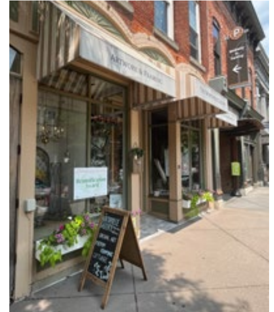
Triangle-shaped awnings that fit above each window and the building's entrance are appropriate. Photo by KDG, 2023.
