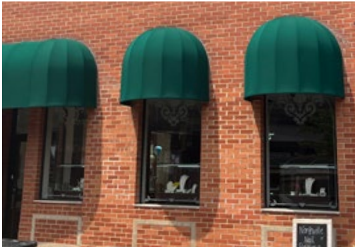
The installation of backlit bubble awnings on historic commercial resources is not appropriate as these types of awnings were not historically used. Photo by KDG, 2023.
