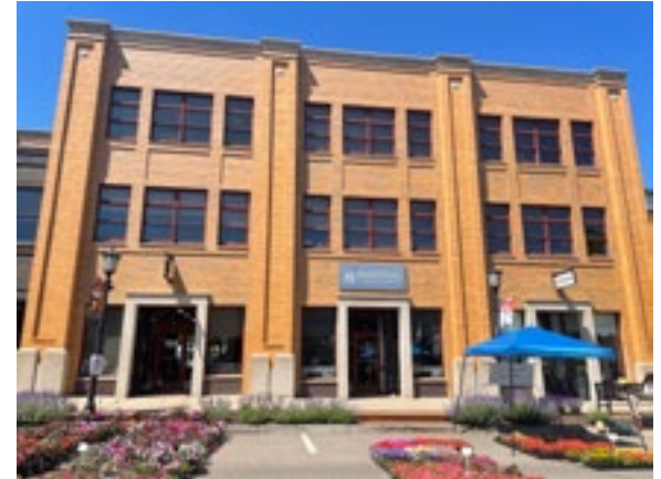
A great example of new construction in Northville that uses compatible design concepts to integrate into the existing historic fabric of the district. Photo by KDG, 2023.
