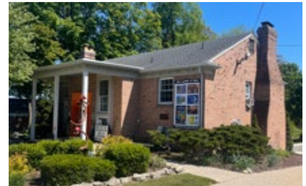
The Scout Building on W. Cady Street is an example of the Colonial Revival style. Photo by KDG, 2023.
