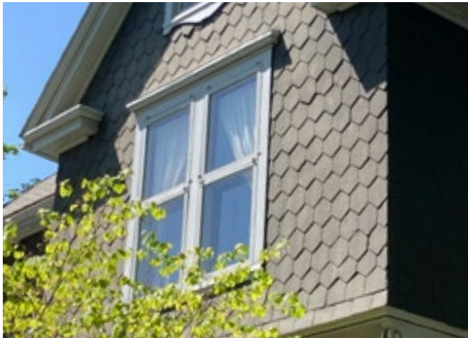
Inspect masonry wall materials on a regular basis and re-secure loose slate tiles when necessary. Photo by KDG, 2023.
