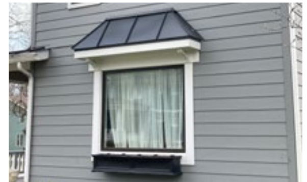
Fixed windows with no mullions or muntins are not appropriate unless the house historically had windows of this type. Photo by KDG, 2023.
