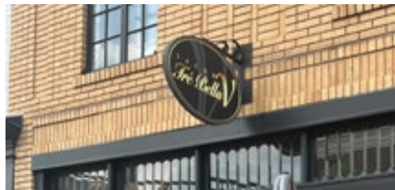
The hanging sign pictured above is located in a historically appropriate area of the building's facade. Photo by KDG, 2023.
