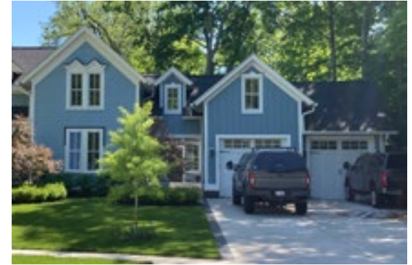
The materials and details on the garage addition are complementary to the historic portion of the house without. Photo by KDG, 2023.
