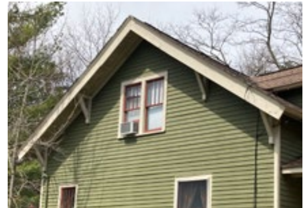
Knee braces are an important decorative feature on Craftsman style houses. Photo by KDG, 2023.
