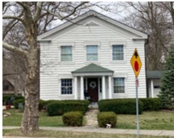
One story entry porches are common on Greek Revival style houses in Michigan. Photo by KDG, 2023.
