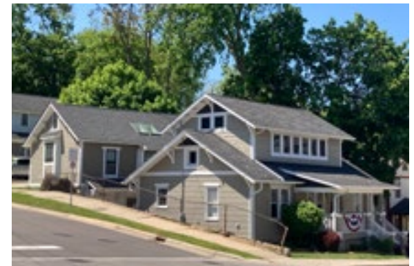
While the materials and details of the second-story addition and outbuilding at the rear are complementary to the historic building, the scale and hierarchy of the new construction is not appropriate in the historic district. Photo by KDG, 2023.
