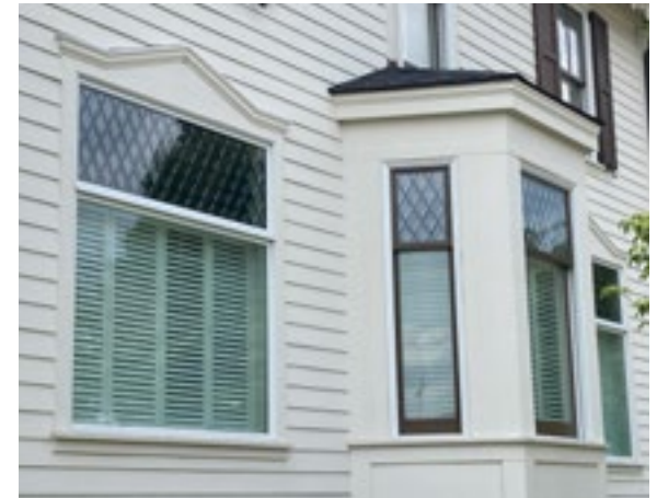
Adding modern (or salvaged) beveled lite windows can create a false sense of history when applied to a building that never historically had windows of this type. Photo by KDG, 2023.
