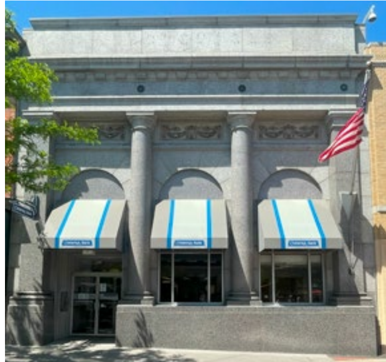
The symmetrical façade, Ionic engaged columns, and modillioned cornice are indicative of the Neoclassical style. Photo by KDG, 2023.
