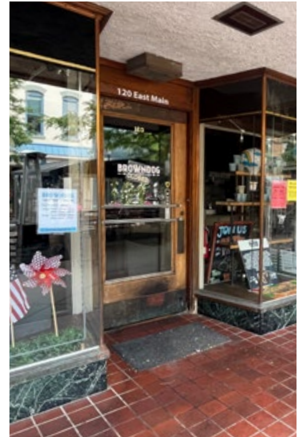
Following the Secretary of the Interior's Standards will help ensure owners, architects, and developers retain buildings and features that contribute to the character of the local district. Features like these large plate glass windows would be difficult or impossible to replace. Photo by KDG, 2023.
