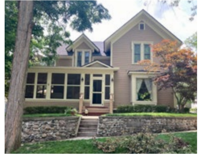
Historic site features like this rubble rock retaining wall should be preserved and maintained. Photo by KDG, 2023.
