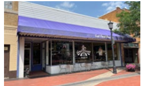
It is likely that the commercial building above was originally clad in masonry. Covering masonry materials with vinyl siding is not appropriate. Photo by KDG, 2023.
