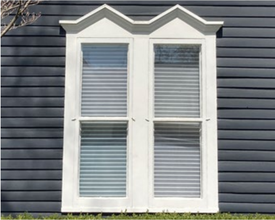
Installed and used properly, storm windows like those pictured above help historic windows conserve energy. Photo by KDG, 2023.
