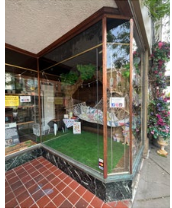
The historic metal storefront system illustrated above should continue to be maintained and preserved. Photo by KDG, 2023.
