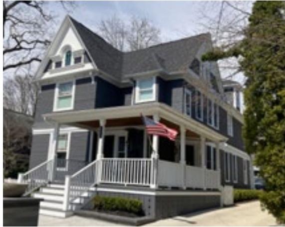
This Queen Anne style home has a steeply pitched roof and a Palladian window at the third story, both of which are associated with this style. Photo by KDG, 2023.
