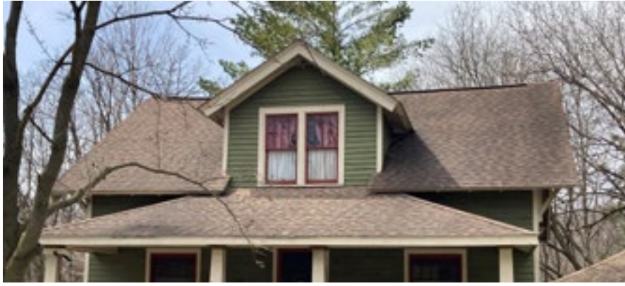
Asphalt shingles are the most common roofing material in the historic district. Photo by KDG, 2023.
