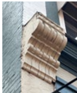
Wood architectural ornament on one of Northville's historic commercial buildings. Photo by KDG, 2023.
