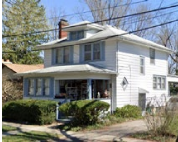
The centrally placed dormer at the attic level and the three-over-one windows are common features in Prairie style houses. Photo by KDG, 2023.
