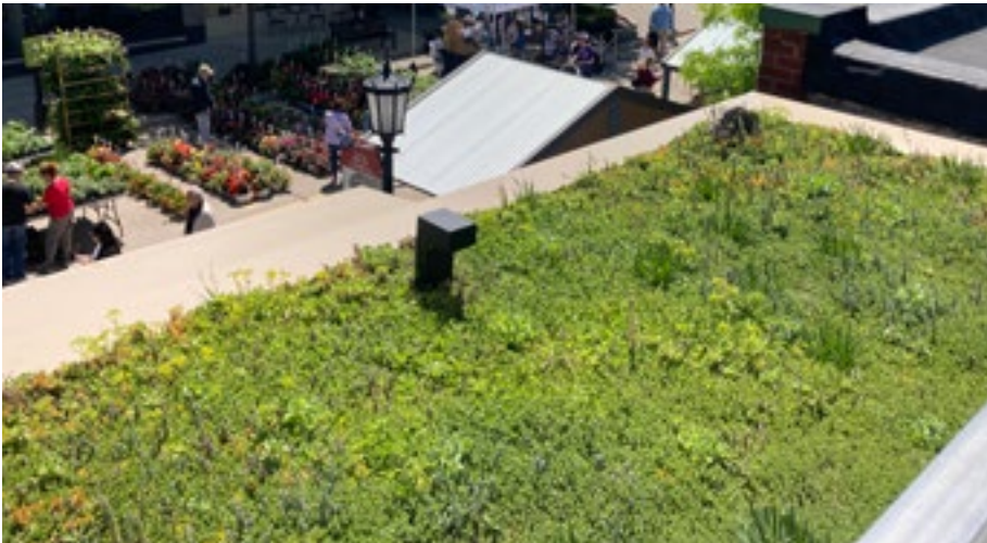
One method to make a historic building more sustainable is incorporating a green roof. However, green roofs require intense study to ensure the building can support the additional weight, water retention, and other needs. Photo by KDG, 2023.
