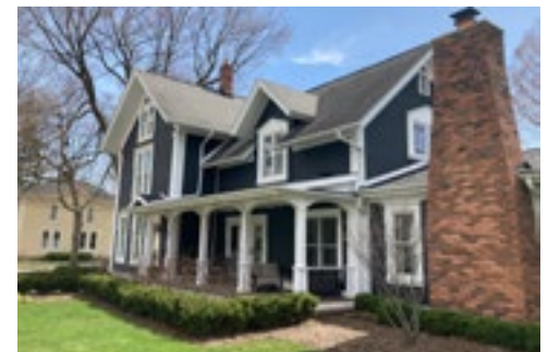
This house was originally built as a one-story structure. In 1888 the second story was likely added. This is another example of a building that, although altered from its original design, has gained significance over time. Photo by KDG, 2023.
