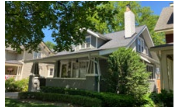
Porches are an important feature on many historic houses and should be retained and preserved. Photo by KDG, 2023.
