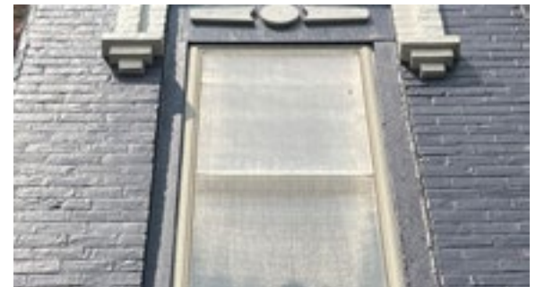
The installation of window screens as pictured on historic commercial building windows is not appropriate. The color of the screening and framing, and placement within the window opening obscures the window behind the screen and draws unnecessary attention to the screens. Photo by KDG, 2023.
