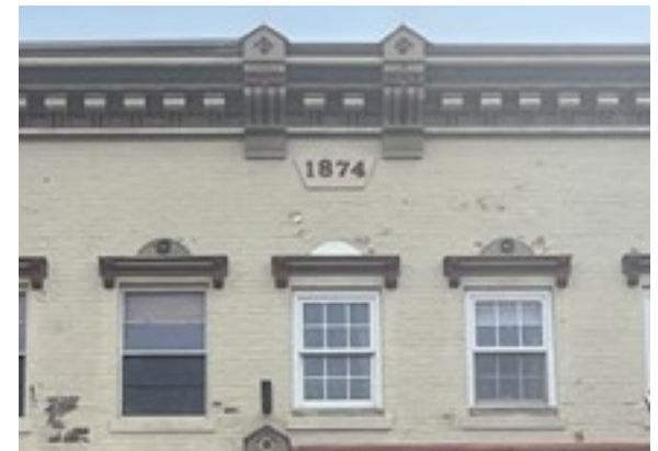
The bracketed cornice and window hoods indicate the Italianate style on this commercial building. Photo by KDG, 2023.
