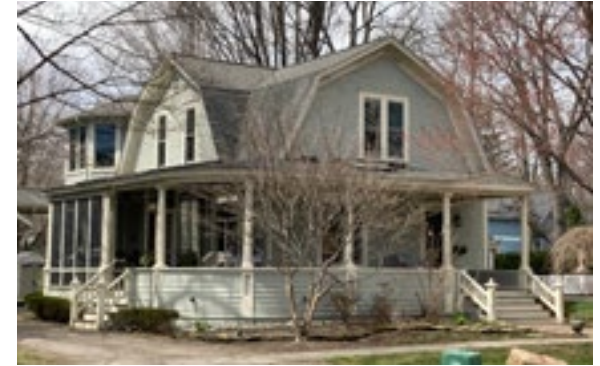
Dutch Colonial is a sub-type and is easily identified by its gambrel roof. Photo by KDG, 2023.
