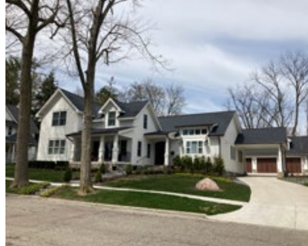
Large outsized additions on the primary façade are not appropriate. Photo by KDG, 2023.
