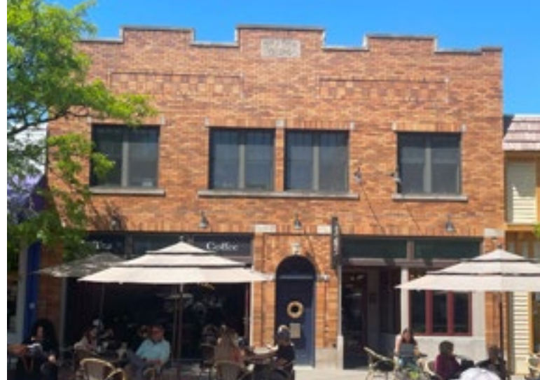
The brick cladding, stepped parapet, and inset basketweave brickwork are key features of the Commercial style. Photo by KDG, 2023.
