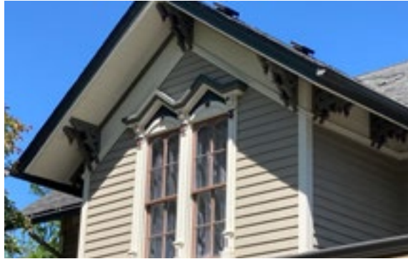
These historic arch-headed windows along with the elaborate window hoods, trim, and molding should be preserved. Photo by KDG, 2023.
