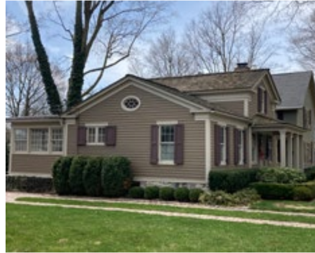
The enclosed porch added to the rear of the house is an appropriate type of addition. Photo by KDG, 2023.
