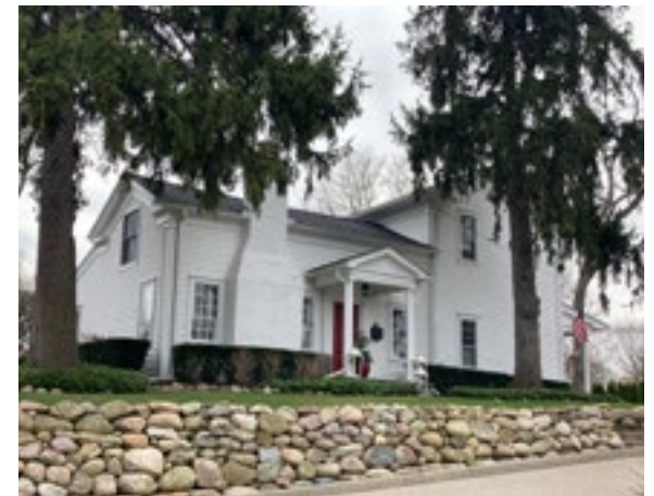
The gable returns, one story entry porch and the pilaster on the corner of this house are all features of the Greek Revival style. Photo by KDG, 2023.
