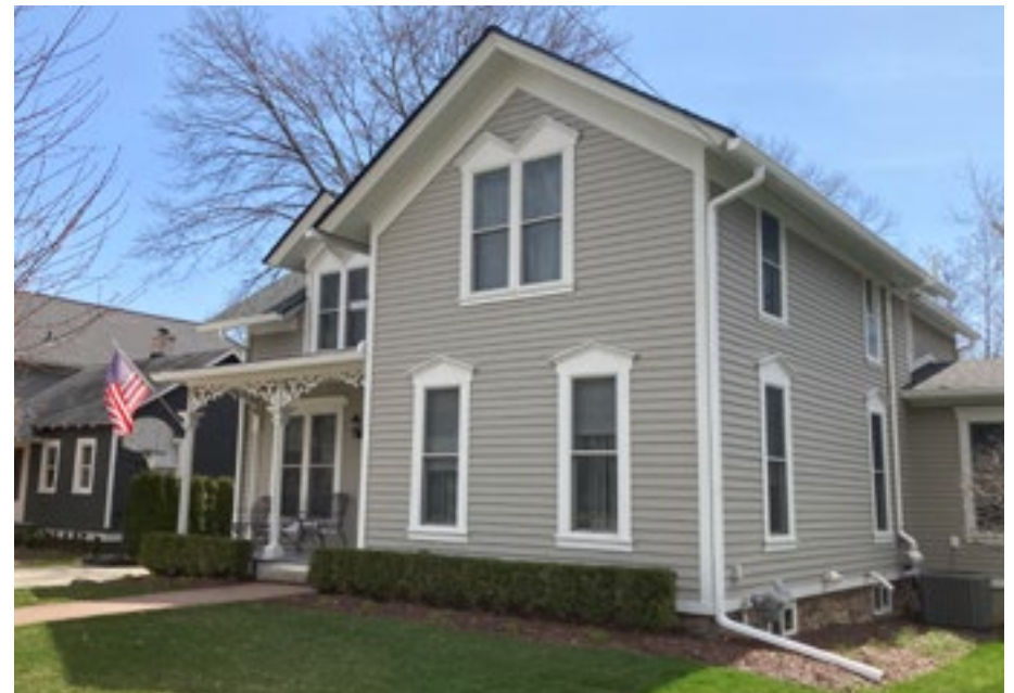
A residential building in Northville's Historic District. Photo by KDG, 2023.
