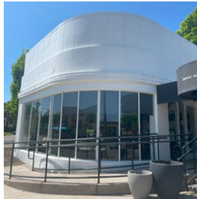
The curvilinear corner of this building and the smooth wall surface are indicative of the Streamline Moderne style. Photo by KDG, 2023.
