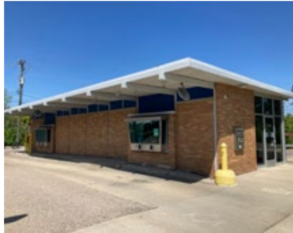
The flat roof, wide overhanging eaves, exposed roof beams, use of brushed aluminum, and fiberglass panels are indicative of Contemporary style buildings. Photo by KDG, 2023.
