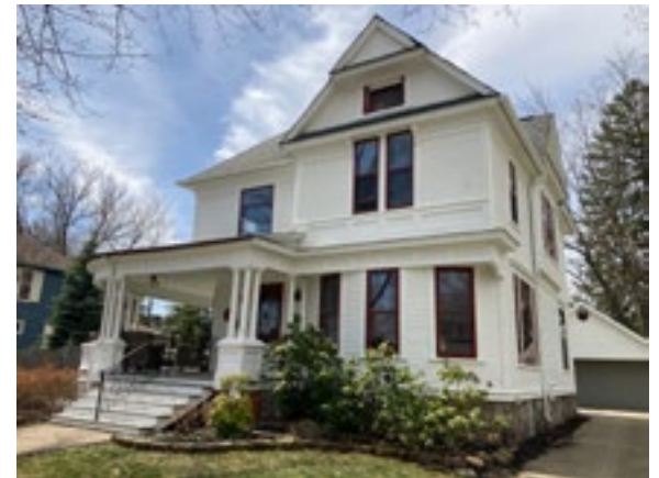
Modern all white paint trends obscure architectural detail that would have been featured and highlighted during the era when this house was built. Photo by KDG, 2023.
