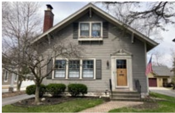
This front gabled Craftsman style house has a low-pitched roof and knee brackets, both typical of the style but the door surround is more classical in style. Not all houses are pure expressions of a particular style; rather architects and designers often mixed and matched stylistic features. Photo by KDG, 2023.
