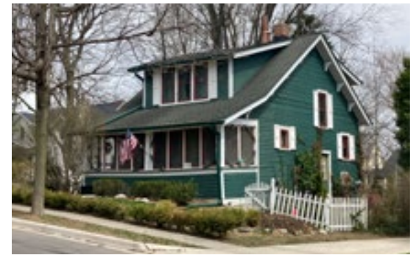
The full width porch, knee brackets, and the centrally placed dormer with a shed roof are all common Craftsman features but the curved trim on the porch is likely a holdover from the earlier Victorian style. Photo by KDG, 2023.
