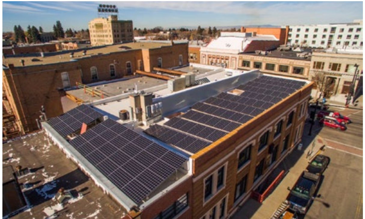
In the example above, solar panels are located on the flat roof of the historic commercial building and are hidden from view by the masonry parapet. Image courtesy of OnSite Energy.
