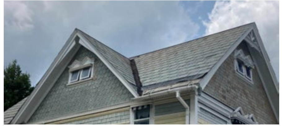
Slate roofing should be retained and preserved. KDG, 2023.
